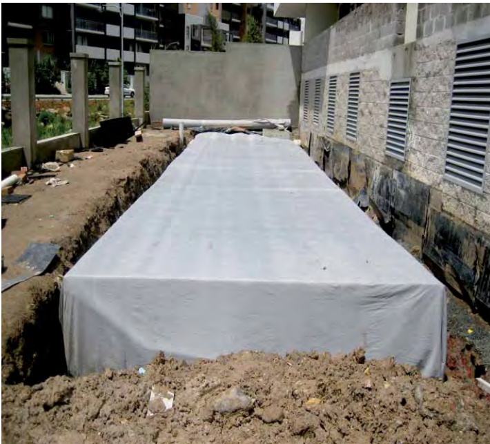
VersiTank® Retention System installed under a landscaped area allows water to be re-used
