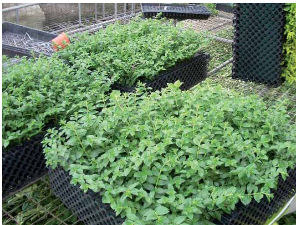
11. Insert plants and allow time for establishment before installing vertically
