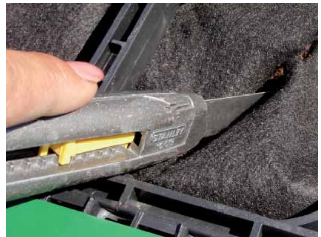
10. Use a sharp knife to slit the geotextile
